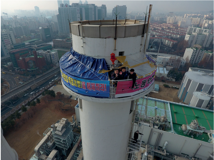
Figure 8 Sky protest by Finetek workers at Mokdong power plant chimney
